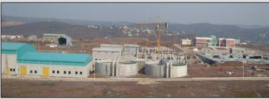
The work includes the design of a complete water treatment plant to provide 720 000 m3 per day of potable water for Istanbul. The water treatment works comprise the process plan and associated buildings. Process design was developed by EMIT, Italy.
